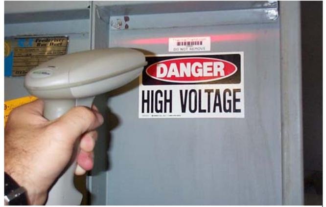
By scanning the bar code the database automatically looks up the equipment so that the thermographer can review the equipment past history.
