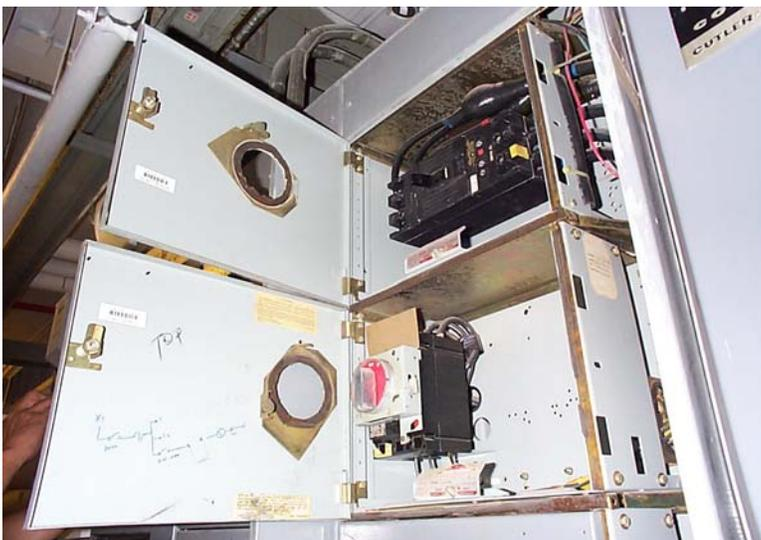
Bar code labels are placed inside the door or next to the equipment to be inspected. This allows for easy tracking of equipment by the database and provides the thermographer the ability to have 100% accountability for what he has and has not tested.
